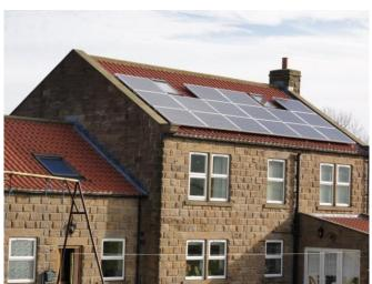
**Issues to consider:-** The system on the barn roof has two inverters, each for 8 panels. Any difference in output will indicate a likely fault. The inverter in the house is in a cupboard and a fault was not spotted for a while. A Bluetooth monitoring system is worth considering.
